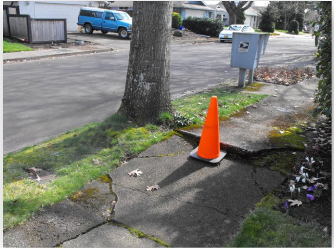
A growing oak tree in a narrow planting strip causing sidewalk damage
