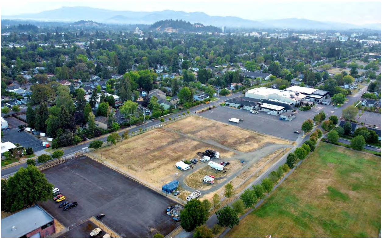
Aerial view from southwest
