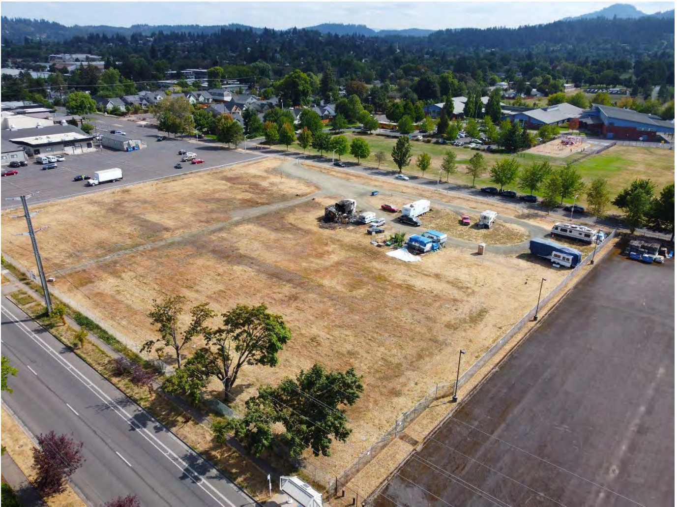
Aerial view from northwest
