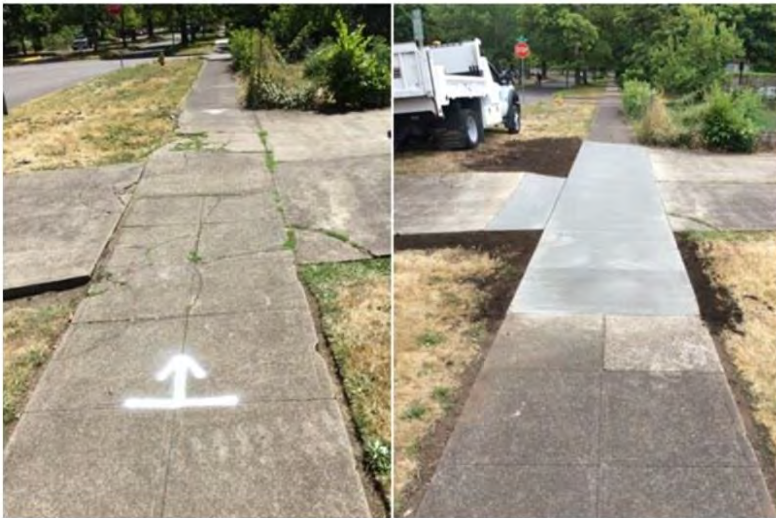
Before and after images of a panel replacement
