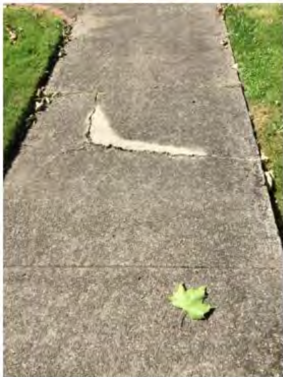
Grinding a minor vertical offset
