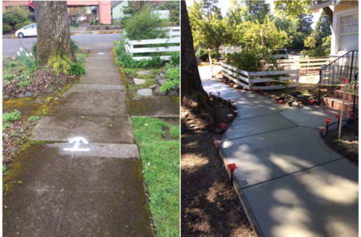
Example of sidewalk rerouted around tree roots
